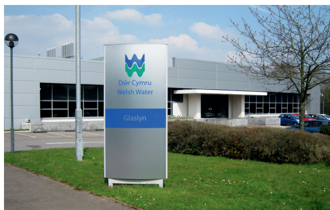
The Dŵr Cymru (Welsh Water) testing laboratory at Glaslyn
